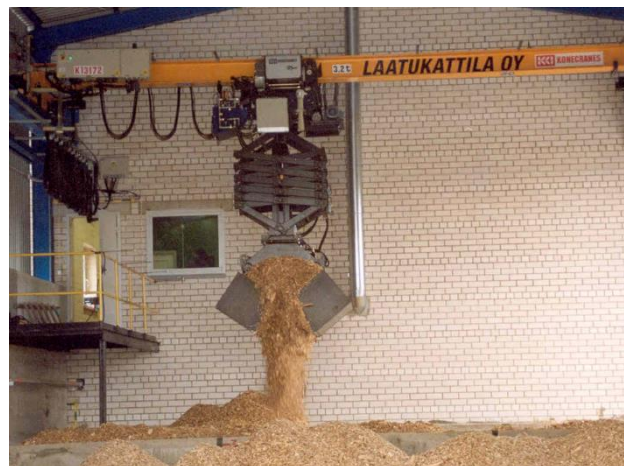
For large fuel storage units (1000 – 3000 m 3 ) Laaturkattila has developed and patented a fuel silo with an automatic crab crane.
