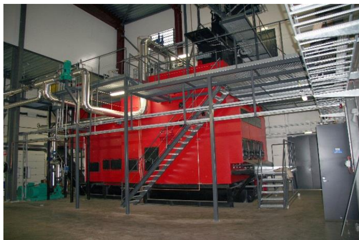
Pansio district heating plant 12 MW Laka Y gasification combustion boilers 5 MW and 7 MW Annual heat production circa 90 GWh
