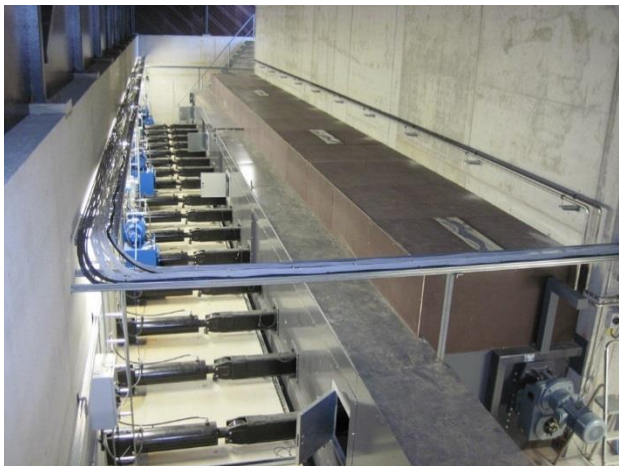
The fuel feed system: cylinders of bar unloaders in a storage, a disintegrator roll and a chain conveyor.
