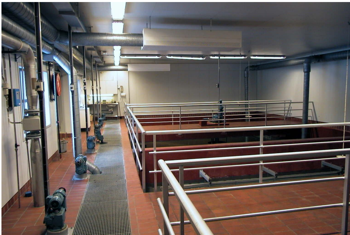
HOLE RENSEANLEGG, SEDEMENTERINGS BASSENG.
